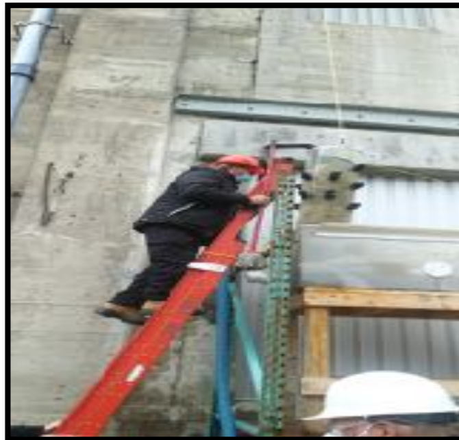
Picture of Wayne Clowater, just finished cleaning the filter.
