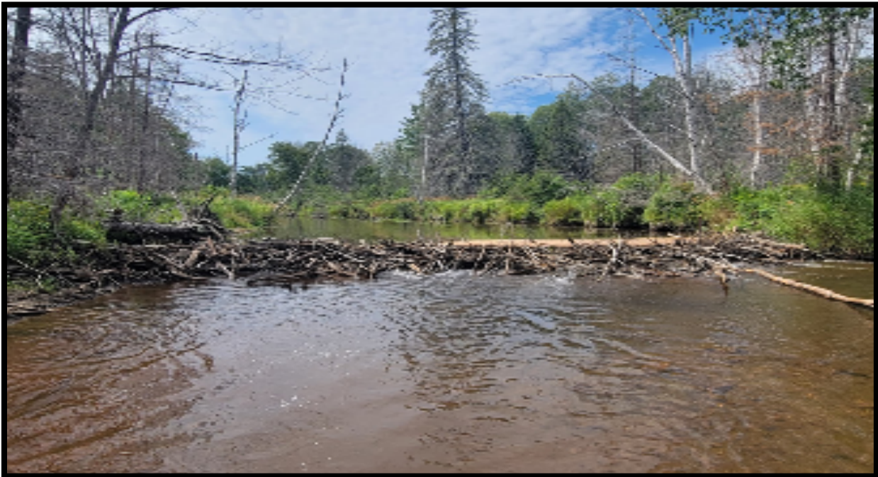
Dam site # 5 (above dam)
