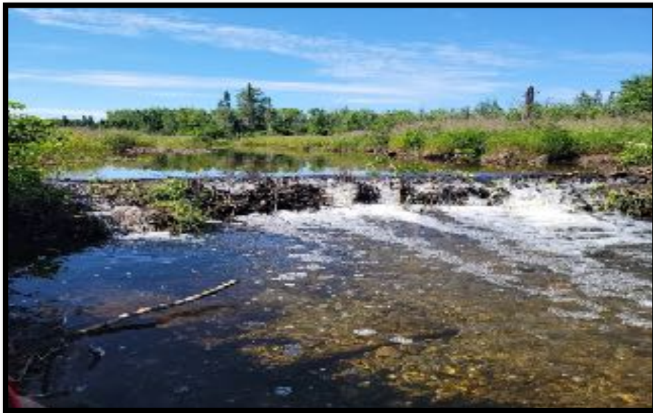
Removed another 4 inches from dam site # 3.
