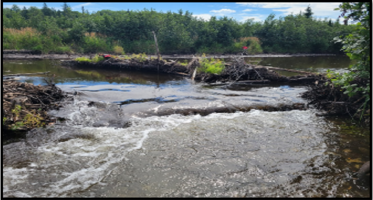
Dam site # 4 completed
